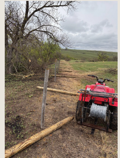
Fence posts laid out ready to be placed.
