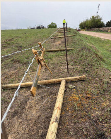
DeWayne Erickson stretching the first line of barbed wire.
