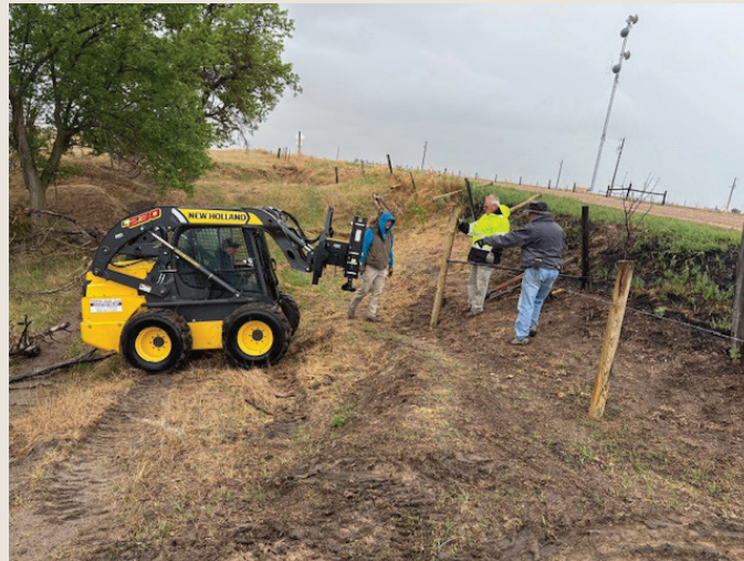
Nick Weber, Ross Nelson, DeWayne Erickson and Walt Rosenbaum working together to set fence posts in the hilly terrain.
