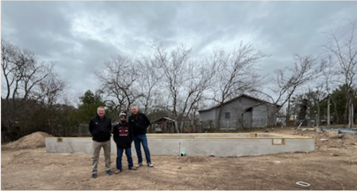
Pete Gnan, Patrick O'Malley and Grant Schmidt stand in front of O'Malley's new cement pad and blocking for his expected new home.
