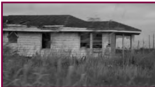
Hundreds of New Orleans homes still wait for rebuilding.
